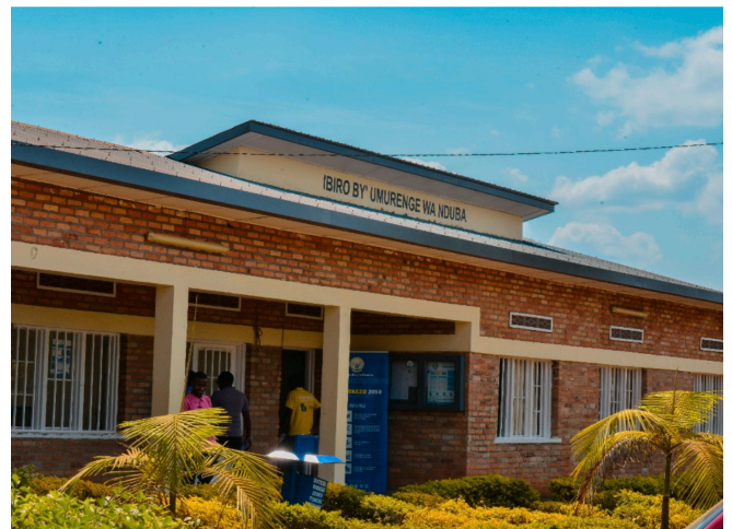
The building hosting the ICT Centre in Kigali, Nduba sector
